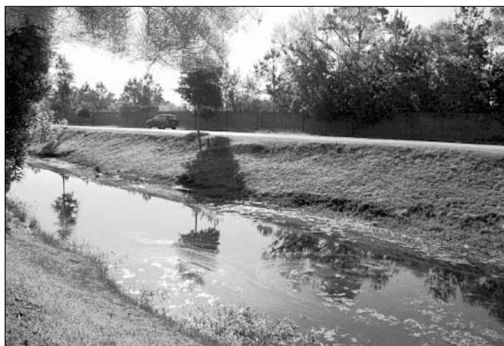
The stormwater retention system at Towne Centre in Mount Pleasant is designed to capture urban runoff such as motor oil, antifreeze, brake dust and fertilizer from impervious surfaces such as pavement. Under current federal guidelines, this pond is considered a man-made wetland.
